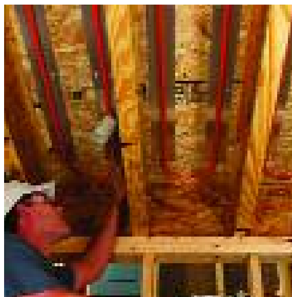
You can install RadiantPEX-AL on the underside of a subfloor, using underfloor plates.
